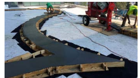
Floradrain® FD 40-E was used as a permanent formwork for the curb and seatwalls.
